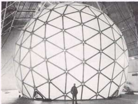
Giant 68-foot rigid radome. This type construction is being studied for domes to 150 feet in diameter
